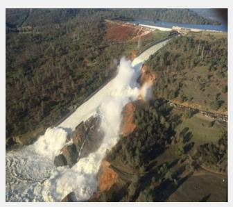
The dam, which is the nation's tallest, remained intact. But the emergency spillway, which guards against the overflow of the dam when water levels are high, was eroding Sunday.
