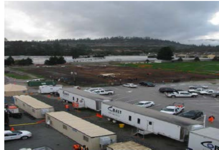
Emergency Base Camp at Scotts Valley in response to winter storms in 2014
